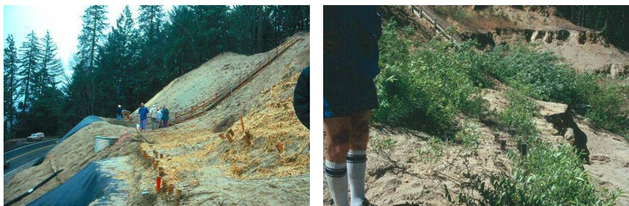
This brush box stabilized the toe of this slide even before the willow became established, and then vegetated the slide.
