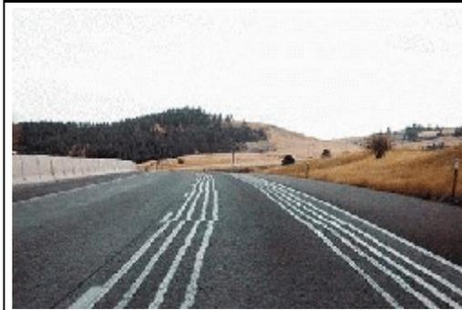
**Copper wires buried in the eastbound right lane of I-84 are designed to heat up and help prevent ice from forming on the road when the temperature is below 28 degrees. ODOT officials emphasize that the system is not an alternative to using chains or traction tires.**
