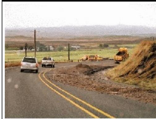
Crews from the Oregon Department of Transportation hauled rock to repair a shoulder along Highway 86 that eroded during a flash flood Thursday afternoon. Debris washed across the highway in two places — at Milepost 17 about 17 miles east of Baker City (above photo), and at Milepost 14. Baker City Herald/Heather Honeywell
